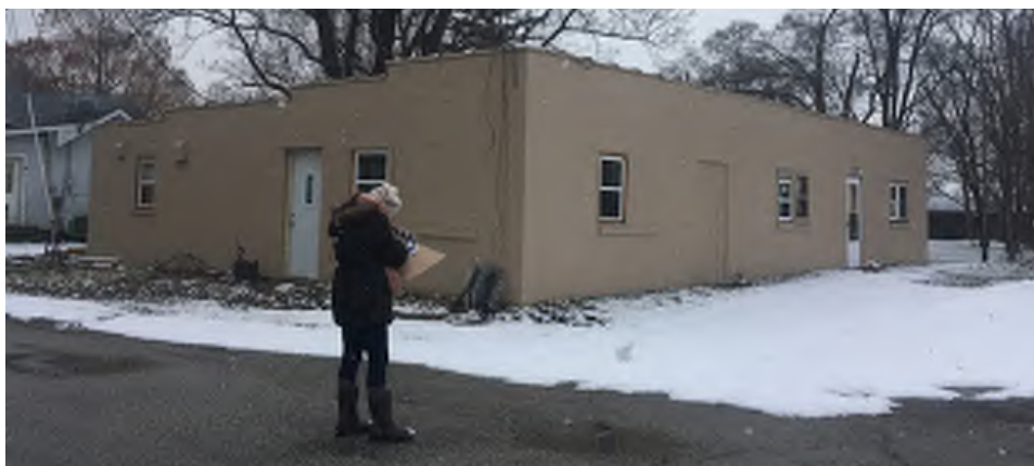
Figure 4.4: Vacant building with potential for use as incubator space.
